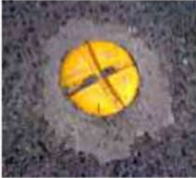
Photo of new sensor imbedded in street pavement.
